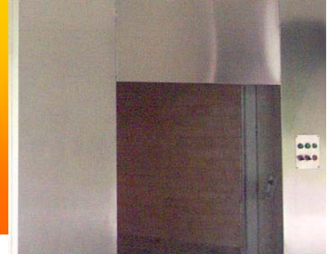
Stainless Steel Cladding
